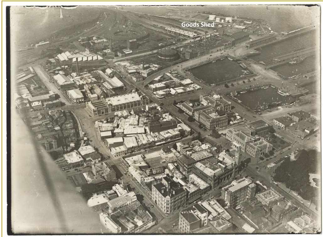
Figure 1: c1920 aerial showing the Goods Shed and study area looking north. Source: Libraries Tasmania Ref: NS892-1-64 accessed 2024.
